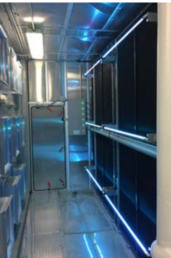
FIGURE 2: UV-C's blue color results from the argon gas in the lamp envelope.
