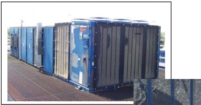
Air Intake Filters mount to the outside of the equipment over the coils where it stops debris from entering – debris is visible, accessible and amazingly easy to clean.
