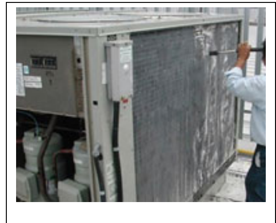
Traditional coil cleaning methods utilize cleaning chemicals and power washers which generates run-off that can enter storm sewers or run off onto the ground.
